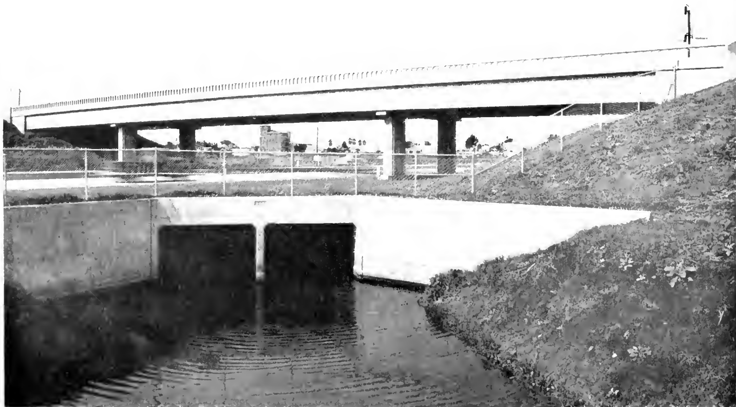
Looking westerly along reclamation district drainage canal showing double 12- x 13-foot reinforced concrete box passing under the Sherwood Drive Overcrossing
